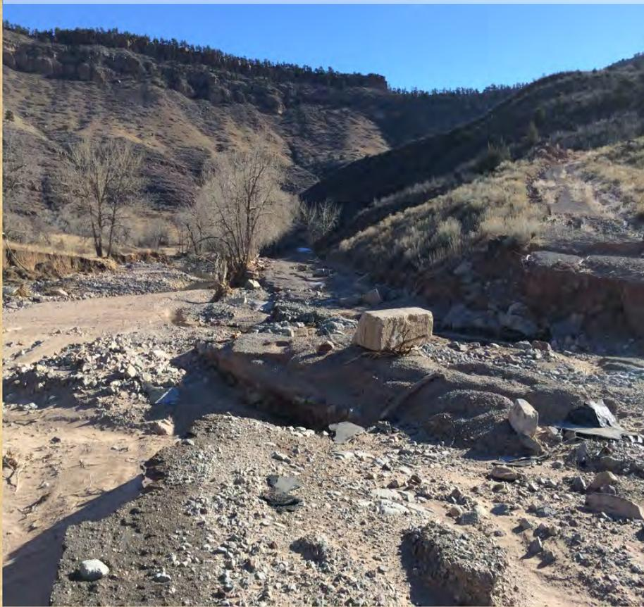
High concentrated flows damaged culverts, caused debris flows across the road and clogged roadside ditches.
