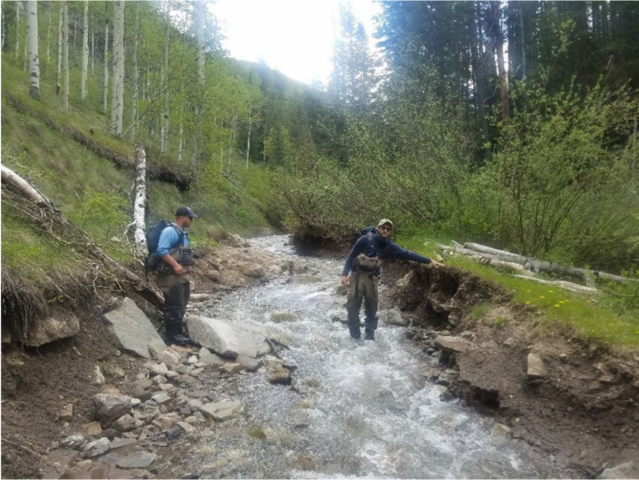
Figure 1. Example of extensive downcutting, erosion, and Wearyman Creek running through the road prism on FSR 708.1 McAllister Gulch, locally known as Wearyman Road. The picture was taken prior to road maintenance completed in Aug. 2022.
